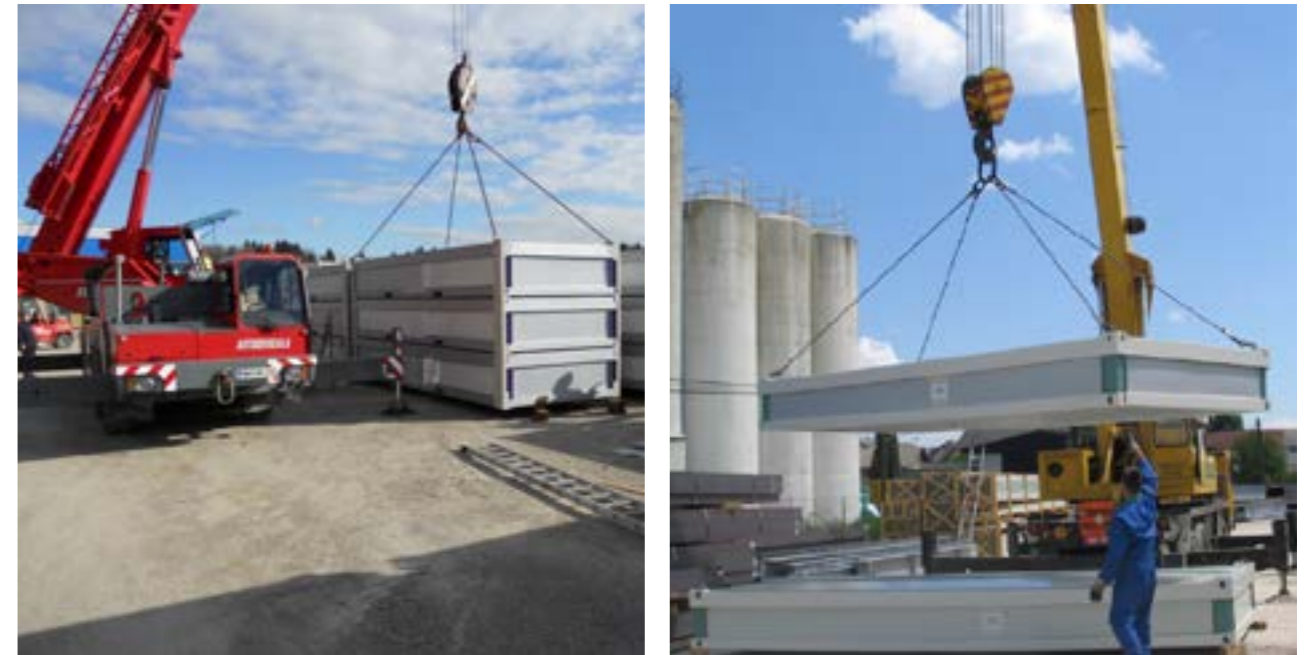
Fig. 1.2: Handling of modular units with crane
