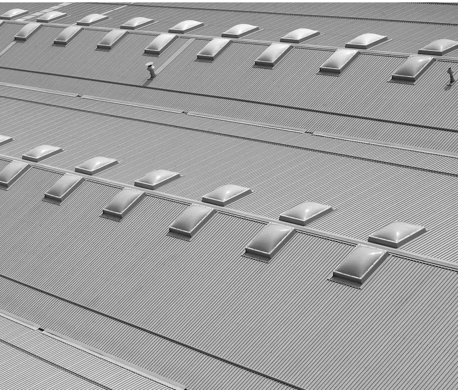
INCLINED ROOF SYSTEM **TRIMOTERM SNV**
